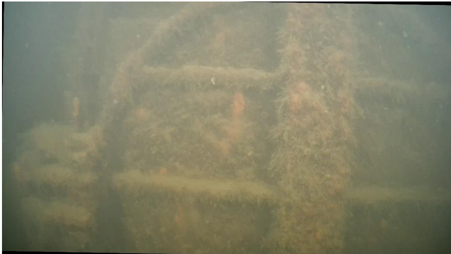
Overview of penstock on left hand external gate
