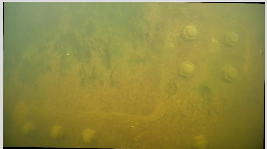
Inspection of bolts on internal gate
