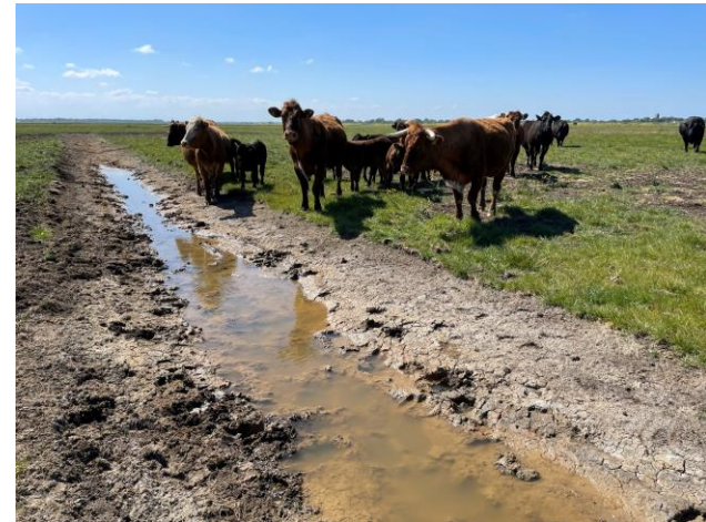
Solar pump and new footdrains funded by CS capital grants – Haddiscoe Island, Norfolk
