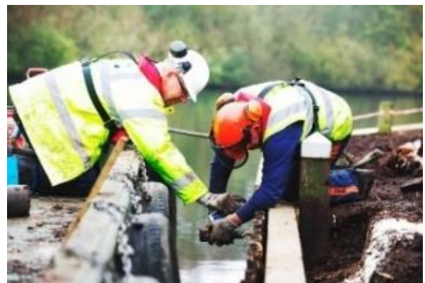
BA Operations technicians refurbishing waterways facilities
