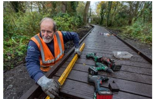
Volunteer working on Hoveton boardwalk repairs
