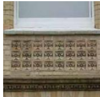
Moulded white brickwork, Station Road
