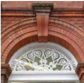
Moulded brickwork and cast iron, Smallgate
