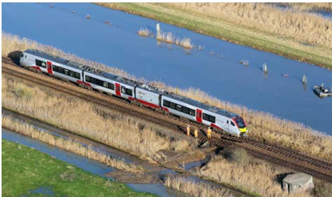
The impact of Storm Malik in January 2022 saw flood water from the River Yare washing away rail track foundations near Great Yarmouth. Mike Page
