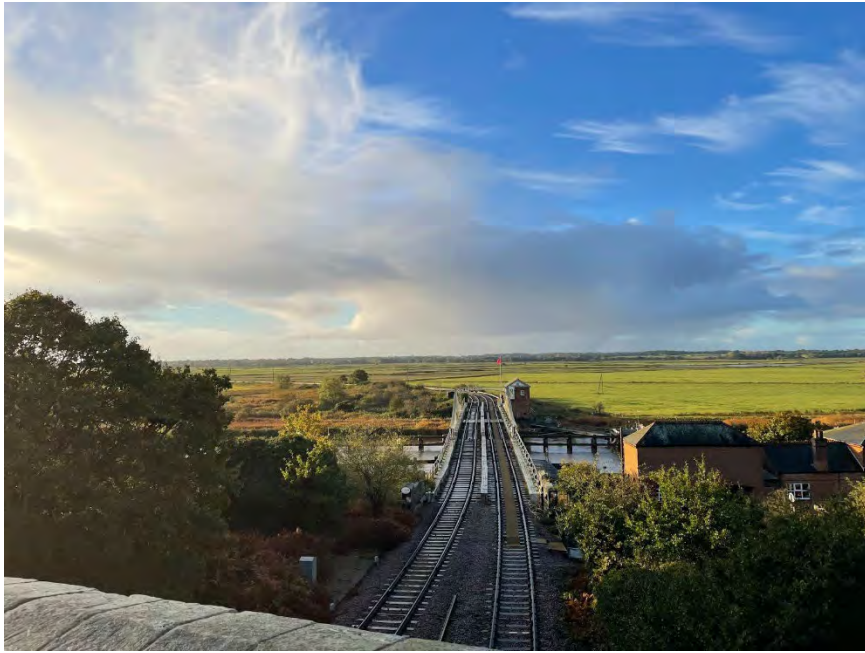
Picture: South from Holly Farm Road railway bridge
