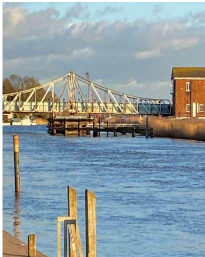
NDHA 3: Reedham Swing Bridge
