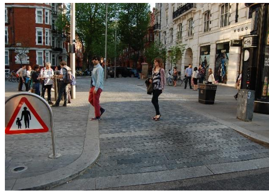
Crossing with similar material to the pavement to act as a traffic calming measure
