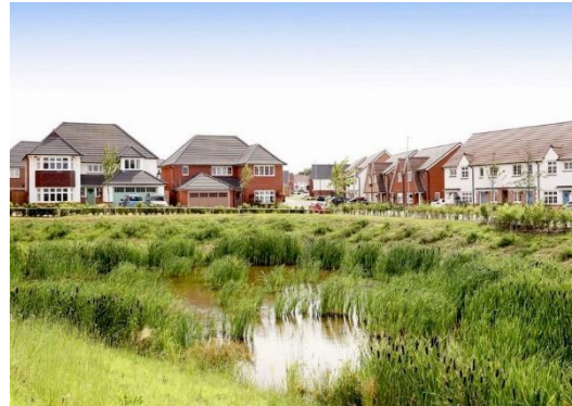
Housing development looking outwards over SUDS for flood mitigation
