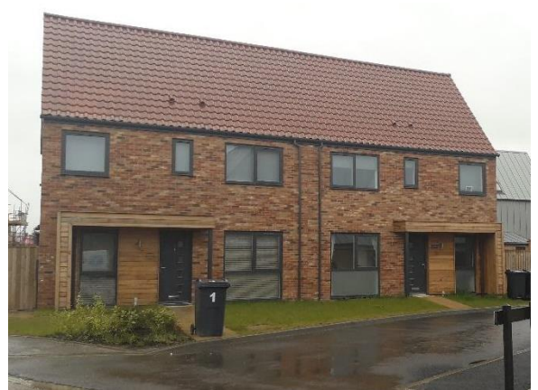
Figure 4.6 Example of a steep-pitched roof on a modern design of property that is not out of keeping with tradition
