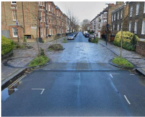
Junction with different surface material and landscaping
