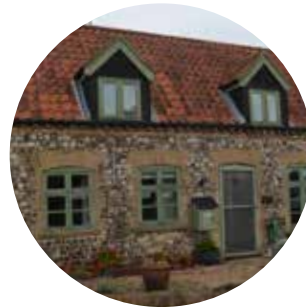
Flint with gable windows
