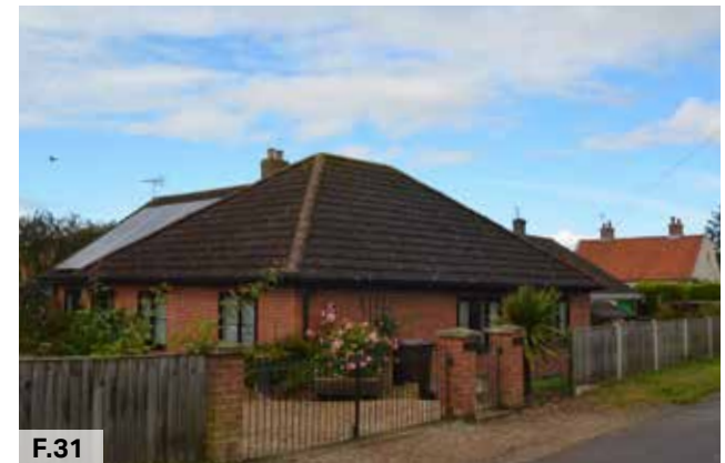
Figure 31: An example of a single-storey dwelling in Reedham with windows on all façades and space in the roof to convert to an additional half storey.
