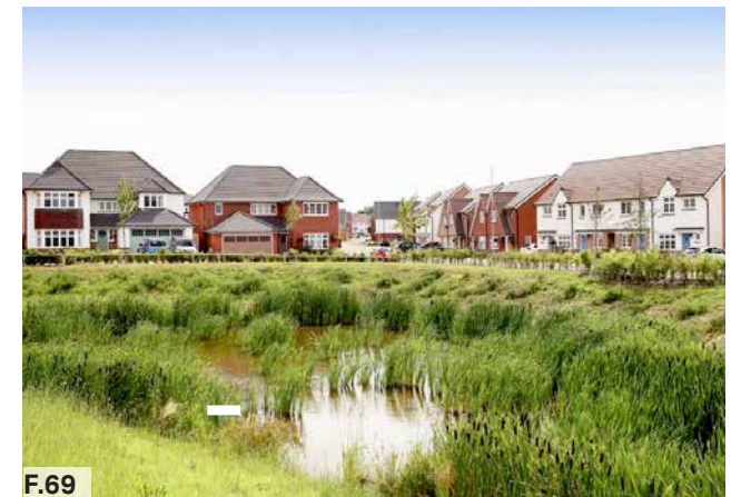
Figure 69: Example of sustainable drainage incorporated into a housing development.
