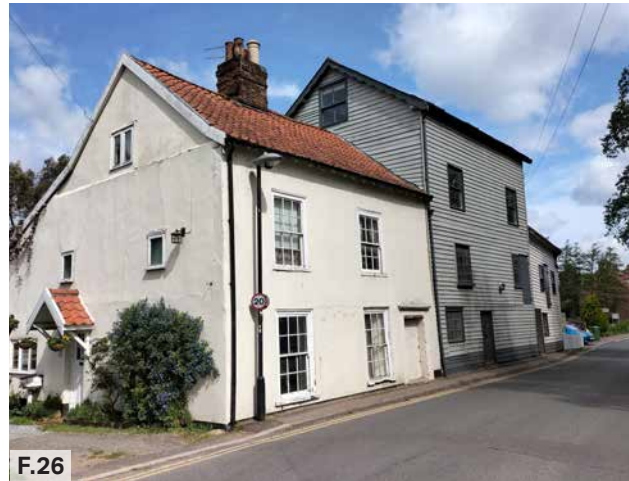
Figure 26: Photo of the Mill, now used for both residential and commercial purposes, with an off white rendered facade adjacent to white-washed weatherboarding.
