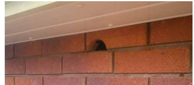
Figure 91: Example of a swift brick under an eave.
