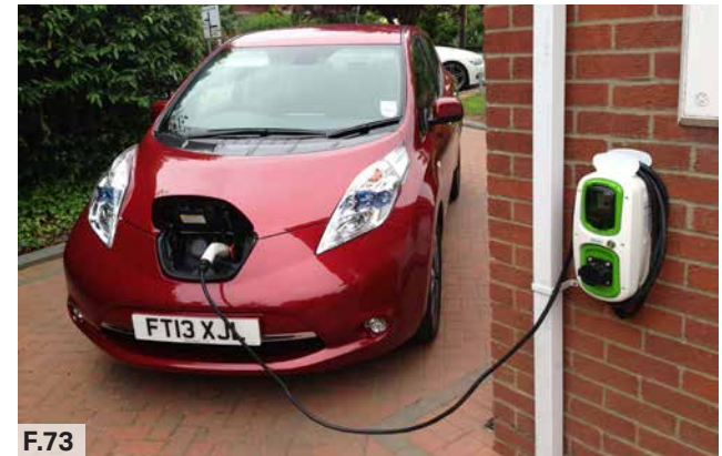
Figure 73: Example of off-road mounted car charging points.
