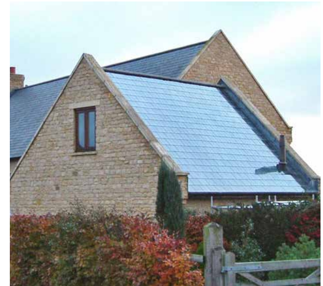
Figure 99: Example of solar panels on a roof in a semi-detached dwelling.
