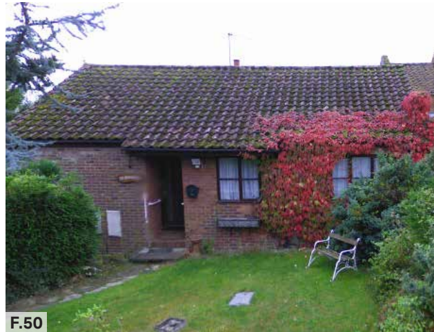
Figure 50: Photo of a single storey dwelling with a red brick facade and clay pantile roof.
