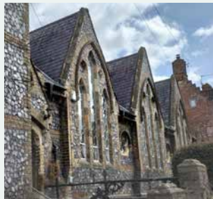
Hood moulded Gothic arched window
