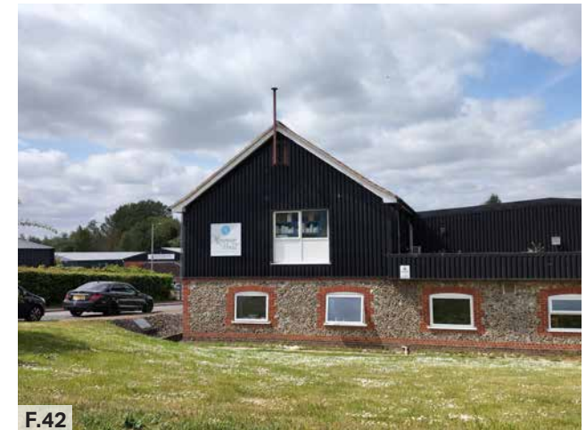
Figure 42: A 2 storey building in the employment character area.
