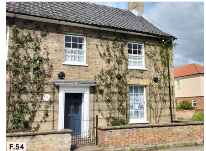
Figure 54: Photo of a 2 storey dwelling in Chedgrave.
