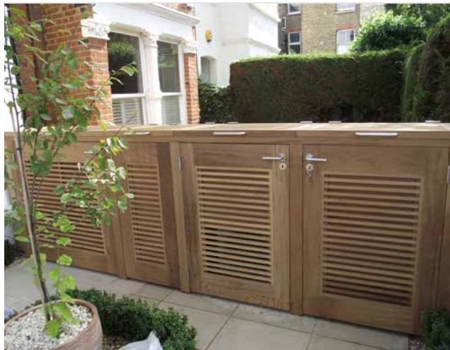
Figure 100: Examples of successful storage design solutions for accommodating bins and bicycles at the front of buildings.
