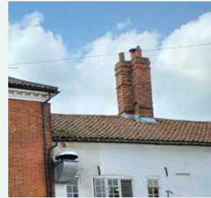
Red brick chimney
