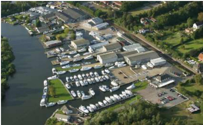
Aerial view of Brooms boatyard (from website)
