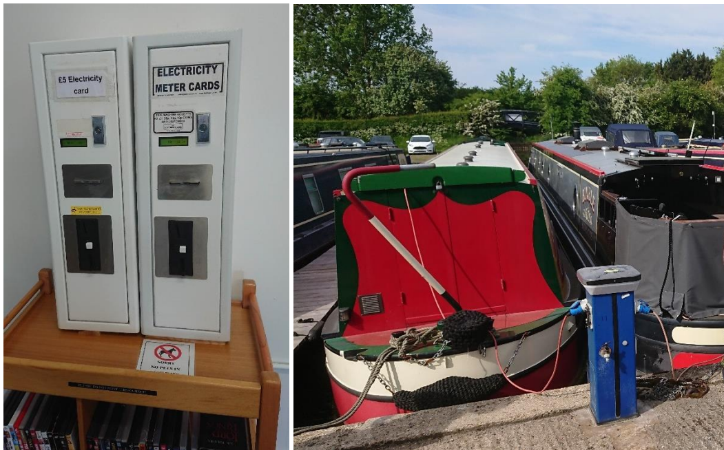
Electricity meter cards dispenser and electricity (and water) unit at Cowroast Marina.
