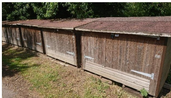
Storage lockers at Priory Marina
