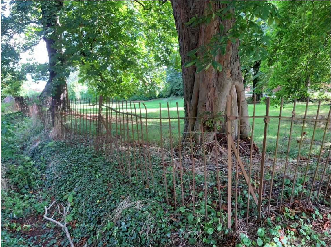
Railings around Sandhole field
