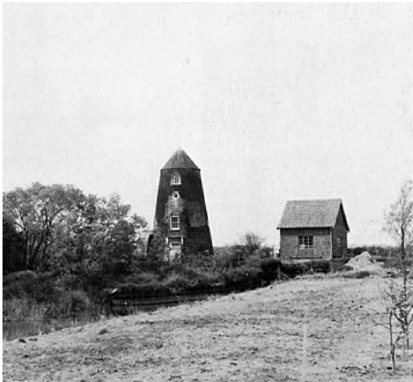
▲ Norton Marsh drainage mill (built in 1863) was built on the south bank of the River Yare just to the east of the mouth of the River Chet and to the south of Reedham Ferry. This photo shows an example of the small red brick buildings constructed to house the pumping gear which was used once electricity had replaced wind as the power source. Recent modernisation of the water management here has meant that the pumphouse is now obsolete and has been demolished. Image courtesy www.norfolk Mills.co.uk
