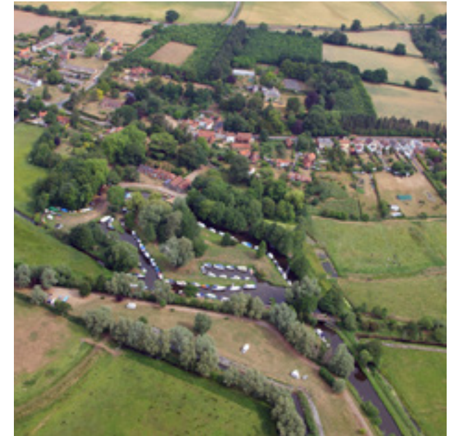
▲ Geldeston is situated on the side of the Waveney valley and connected to the main river by a navigable dyke. Photo by Mike Page.
