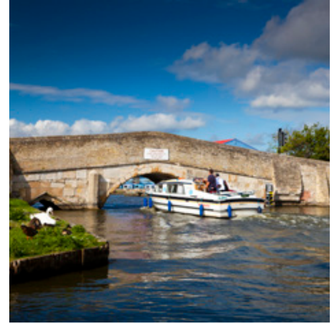
▲ Potter Heigham Bridge – rising water levels over the centuries have limited the size of boat that can pass underneath. Photo by Tom Mackie.
