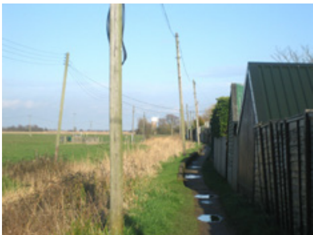
▲ Telephone and electricity cables and poles clutter the landscape and affect the landscape character.
