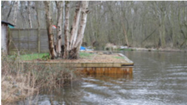
▲ Quay headed frontages installed in the countryside can impact on wildlife habitat by creating an unnatural bank edge.
