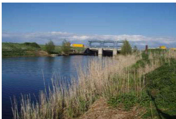
Figure 17: River Delph at the Welmere Lake Sluice
