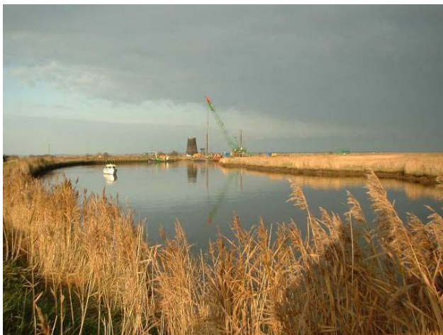
Figure 12: Flood alleviation works at Seven Mile Reach on the River Yare
