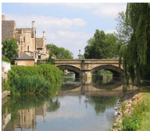
Figure 10: View of the River Welland through Stamford
