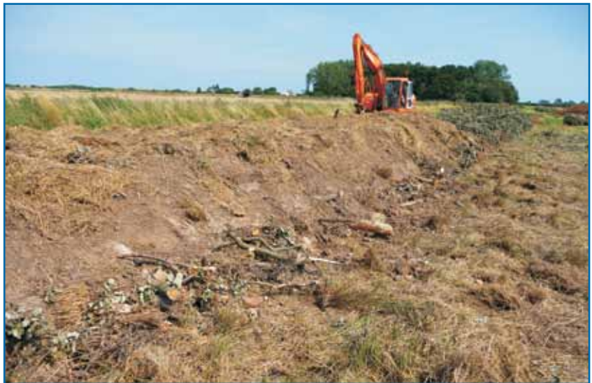
Figure 6 The new reptile hibernacula was specifically located outside but adjacent to the works corridor. It was constructed in layers of locally sourced brush, timber and reed bundles, with topsoil and grass seed applied to develop a dense sward
